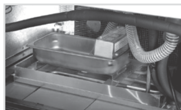
TAC Condensate Heater Pan/Bracket Kit Pictured without back screen.
